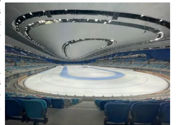
National Speed Skating Stadium (indoor)
