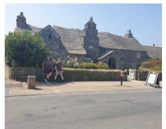
Cornwall - The Old Post Office
